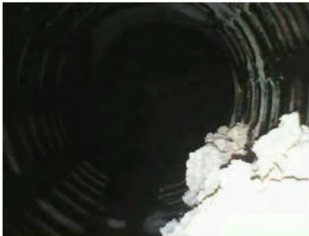
Illustration 79 g06550823 Typical example of DEF deposits in the Selective Catalytic Reduction (SCR) mixer
